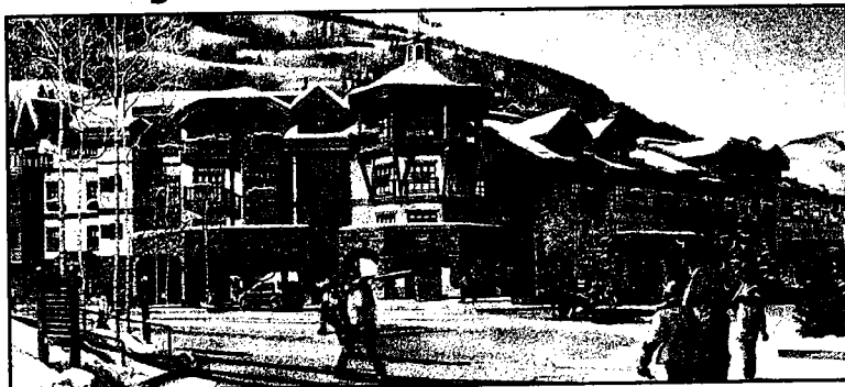
One Willow Bridge Road, a $100 million condominium development under way in Vail, will incorporate the latest in technology.
